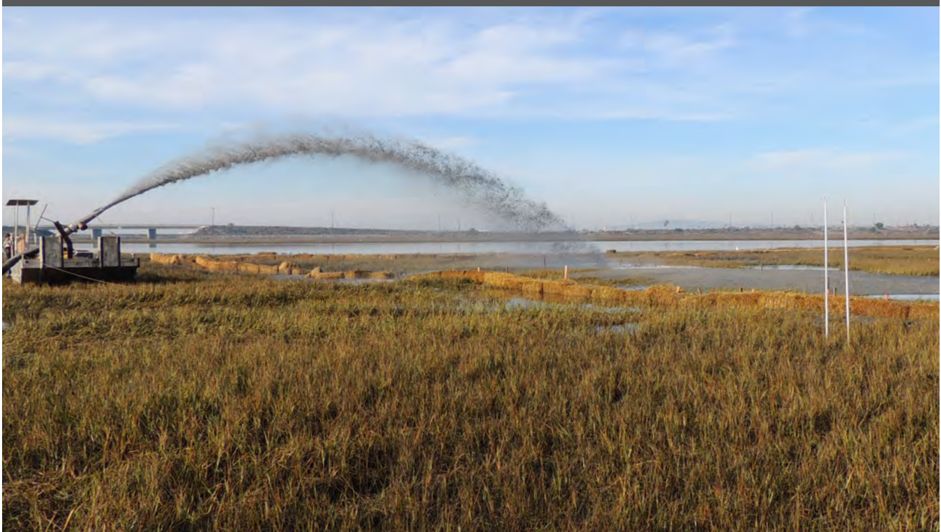
SEDIMENT SPRAYING AT SEAL BEACH NATIONAL WILDLIFE REFUGE • PHOTO COURTESY OF USFWS
