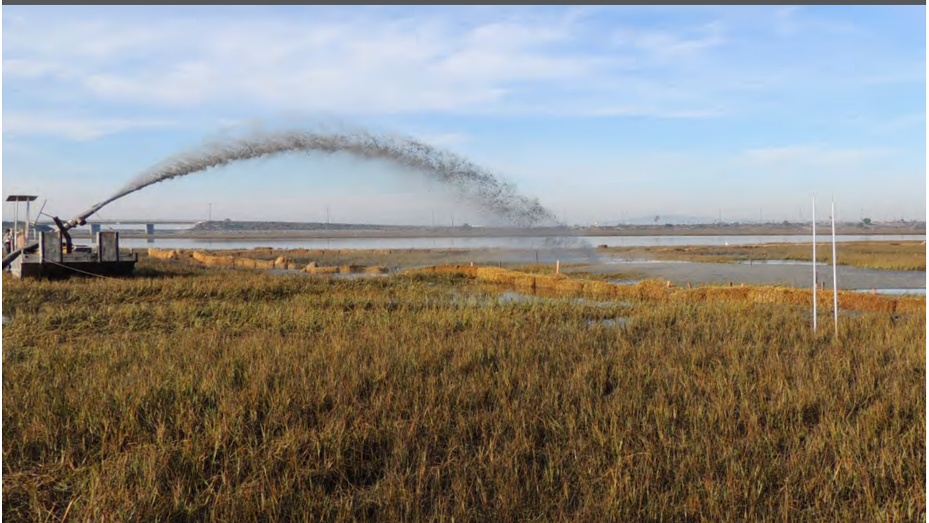
SEDIMENT SPRAYING AT SEAL BEACH NATIONAL WILDLIFE REFUGE • COURTESY OF USFWS
